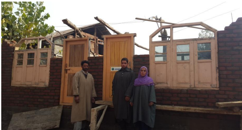
House under Construction
